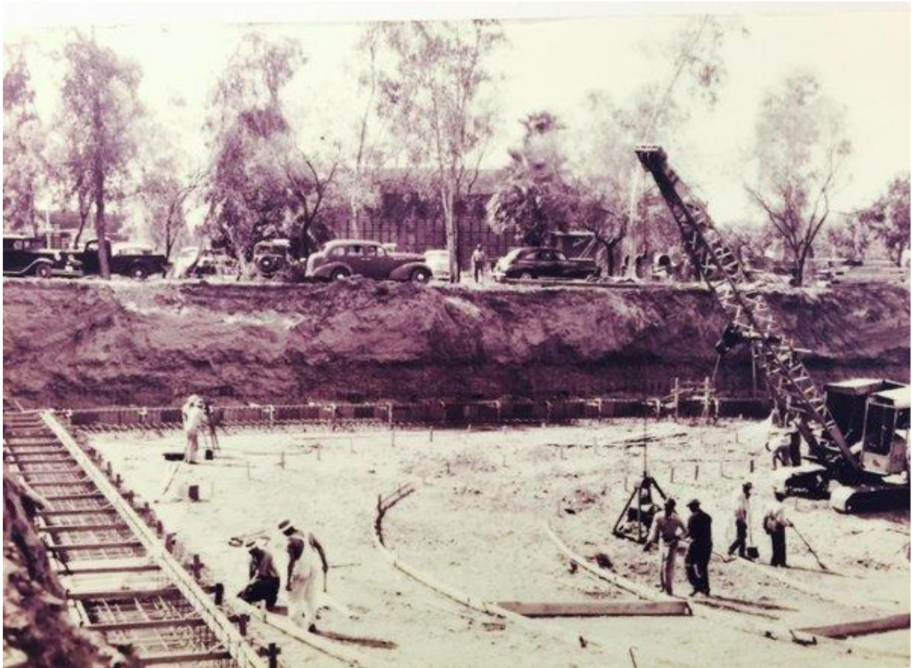
1947 Construction of Clarifier at 23rd Avenue WWTP
