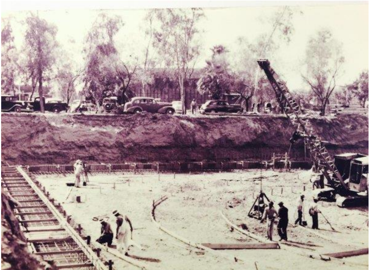
1947 Construction of Clarifier at 23rd Avenue WWTP
