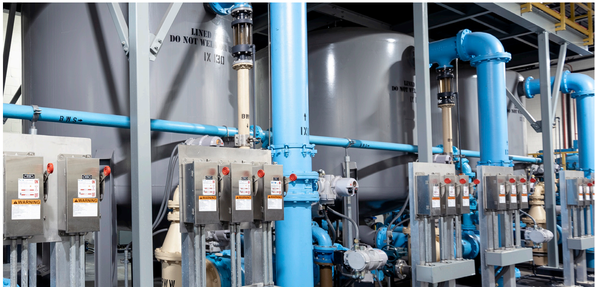
Oasis Water Treatment Plant
