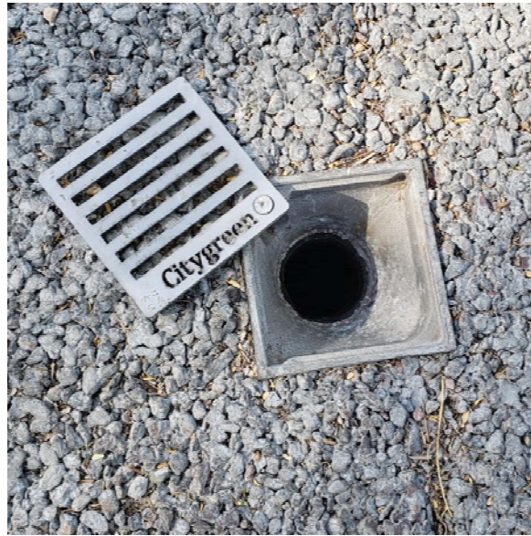
Unclogged drain inlet
