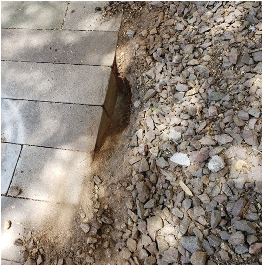
Grouted pavers around edge (header)
