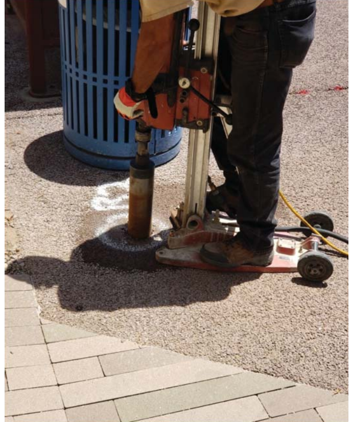
Pavement boring at Central Station
