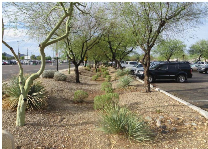
Union Hills Service Bioswale
