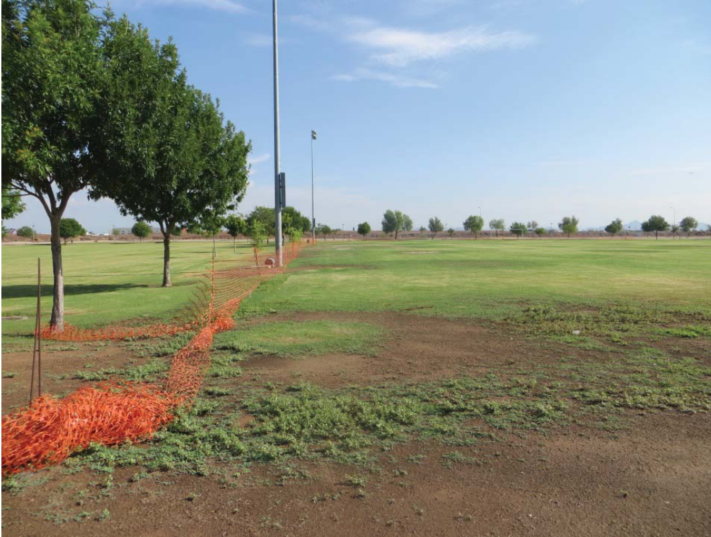
Manzanita Park Turf Bioretention
