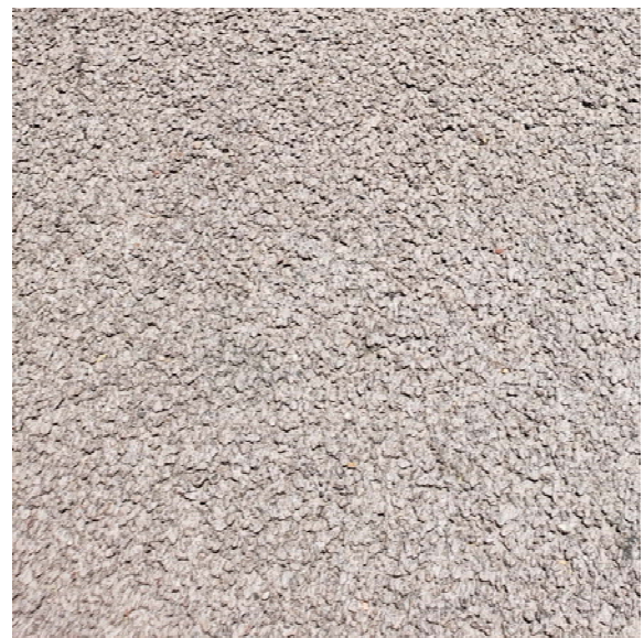
Pervious concrete at Central Station
