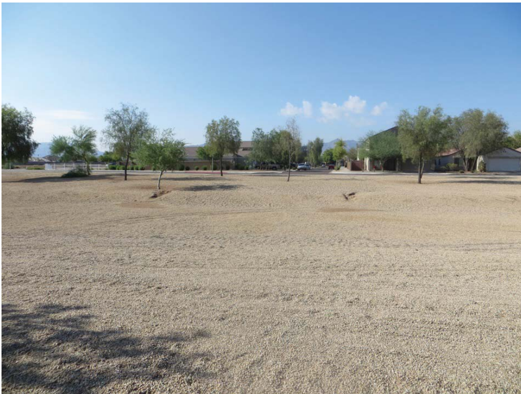
Manzanita Park Decomposed Granite Bioretention
