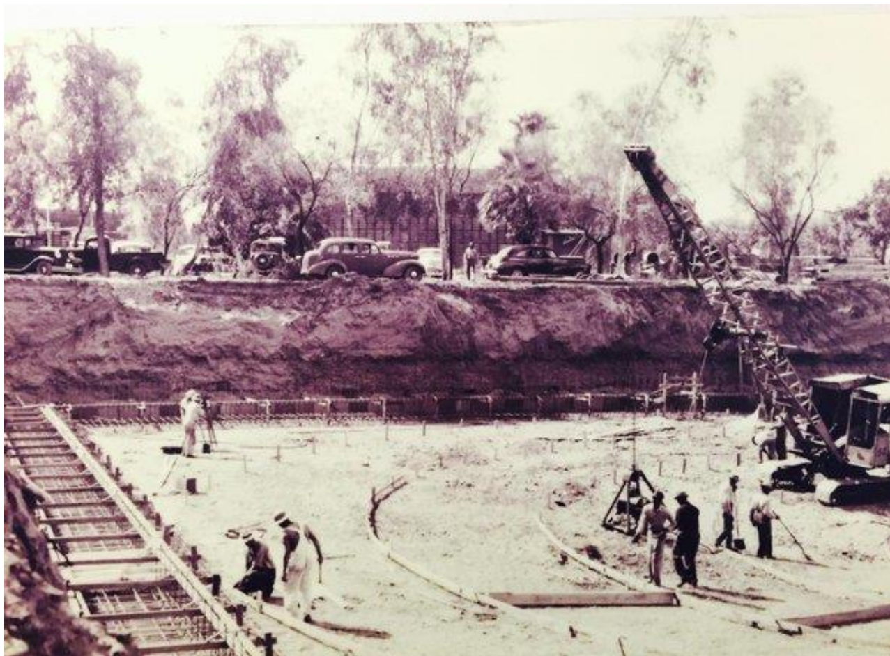
1947 Construction of Clarifier at 23rd Avenue WWTP
