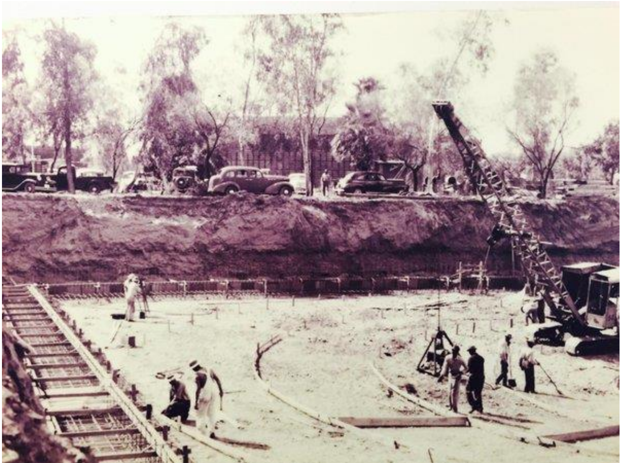
1947 Construction of Clarifier at 23rd Avenue WWTP
