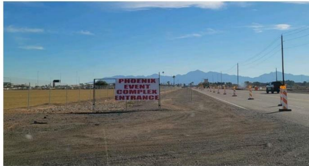
Figure 16: Phoenix Event Complex on 99 th Avenue
