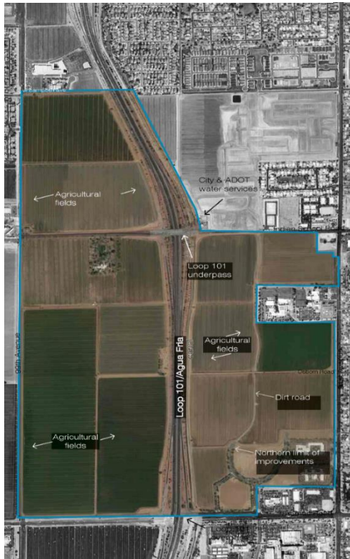
Figure 2-7: Algodón Center Existing Site Conditions
