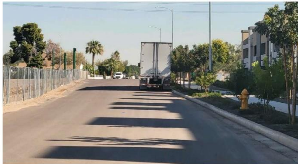
Figure 4: Newly Paved Osborn Road at 91 st Avenue
