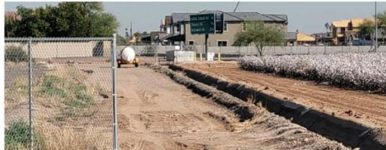
Figure 10: Campbell Avenue Alignment Looking East
