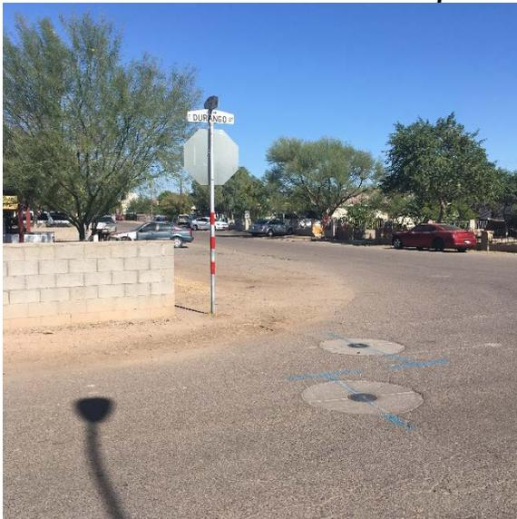
**Photo 63 - ADA Ramp that is not in accordance with ADA Guidelines**
