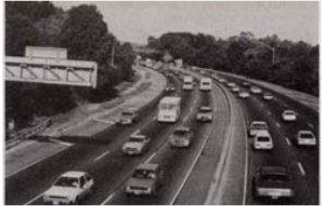
Level of Service D: High-density flow in which speed and freedom to maneuver are severely restricted and comfort and convenience have declined even though flow remains stable.
