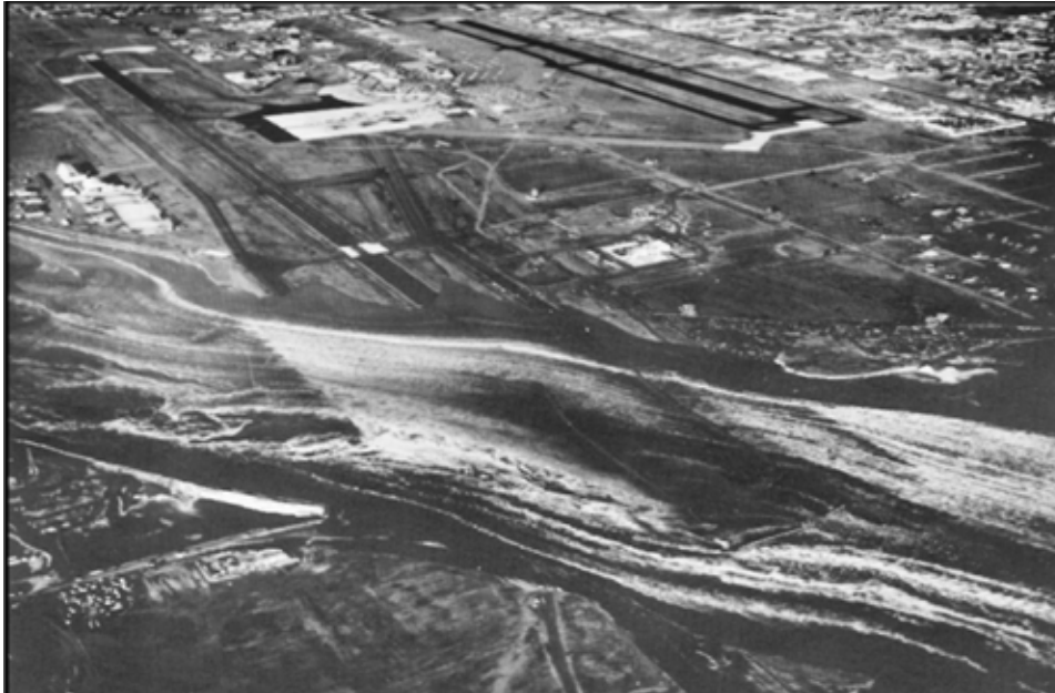
FEMA - Figure 2. Salt River flooding in December 1965 (The 40th Street bridge railing is visible at lower right; flow is from right to left.)
