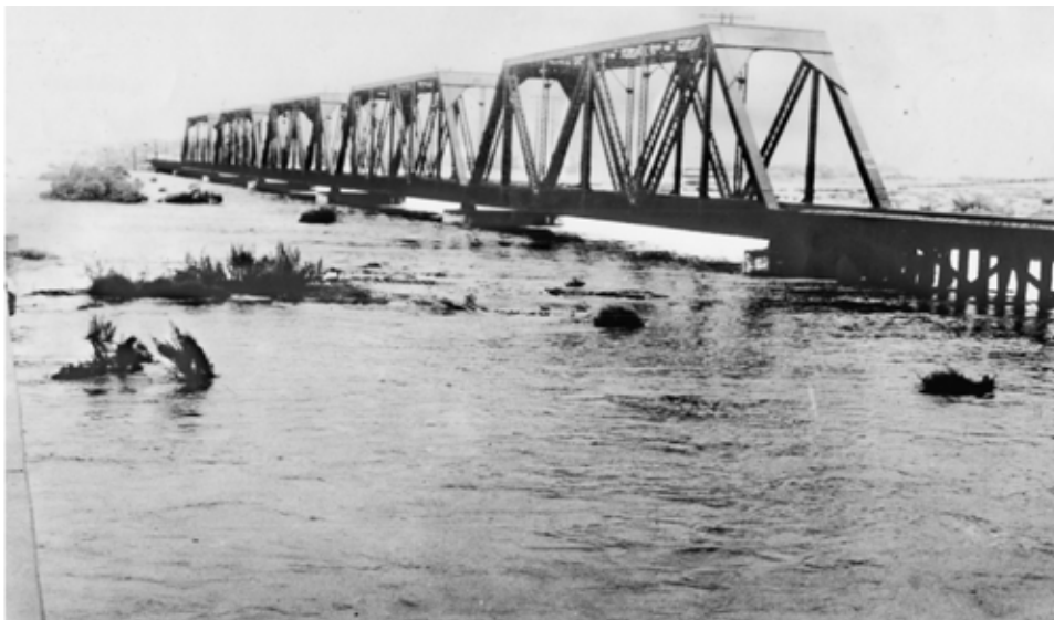
FEMA - Figure 5. Agua Fria River Flooding at U.S. Highway 80 and Southern Pacific Railroad Bridge near the City of Goodyear on December 22, 1965 (Direction of flow is right to left.)
