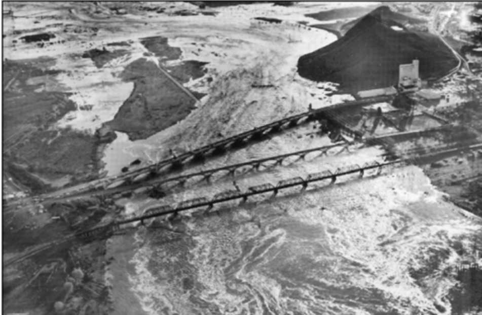
FEMA - Figure 3. The Salt River Bridges in the City of Tempe, looking upstream (The flooded area in the upper center is now developed into athletic fields and parking lots for Arizona State University. Photograph was taken on December 31, 1965.)
