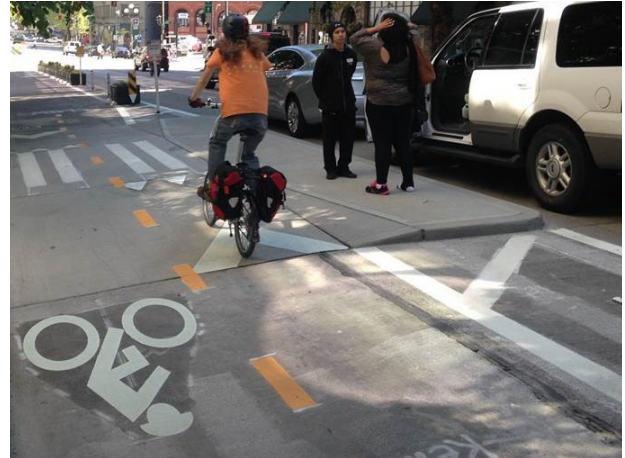
A passenger loading zone allows pedestrians to cross the separated bike lane to access the loading island. These designs should also incorporate truncated domes to alert people walking with vision disabilities of the crossing.
