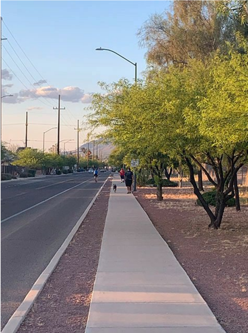
Image: Street with detached sidewalk and shade
