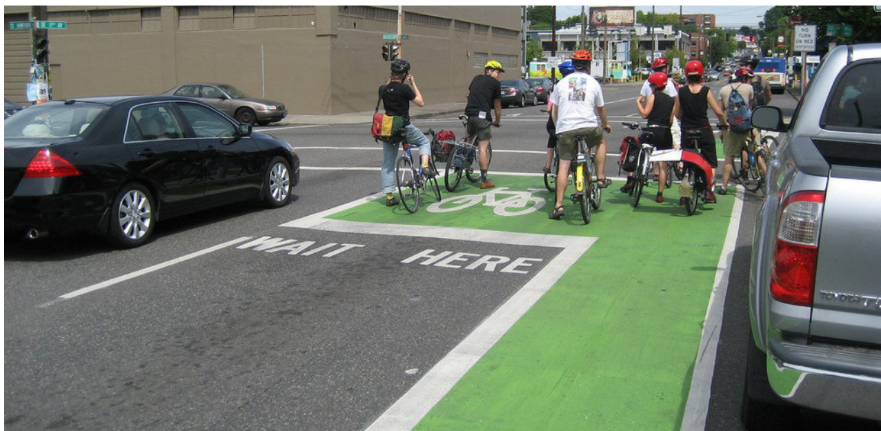
A bike box allows for bicyclists to wait in front of queuing traffic, providing high visibility and a head start over motor vehicle traffic. Photo credit: Marin County.
