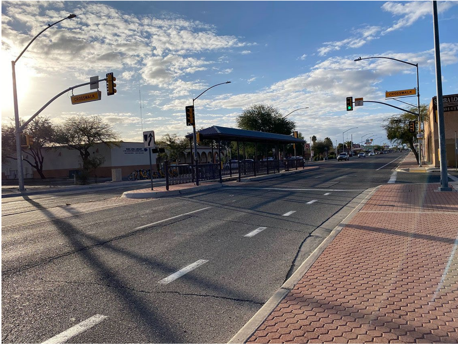
Image: Major street and sidewalk without separation from the roadway (not detached)
