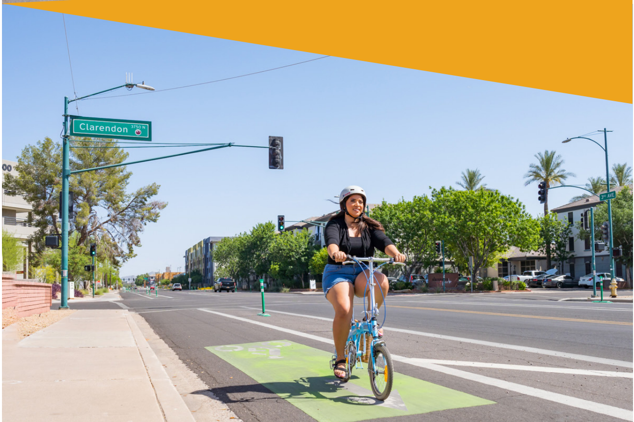
3rd Avenue Protected Bike Lanes with the use of a buffer strip and vertical posts to separate bicyclists from traffic. Source: Maricopa Association of Governments
