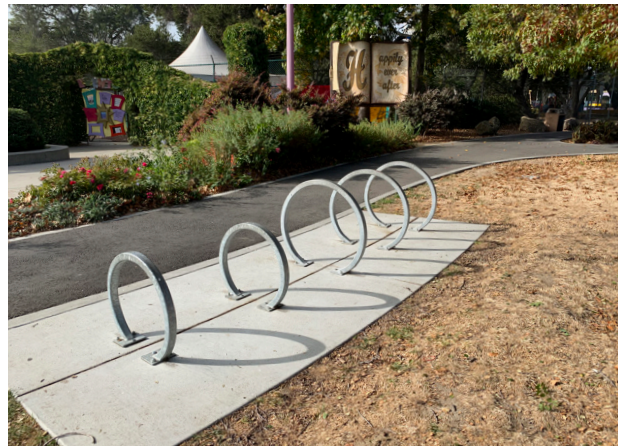
Racks with square tubing, good spacing, and a concrete base likewise offer two points of contact.
