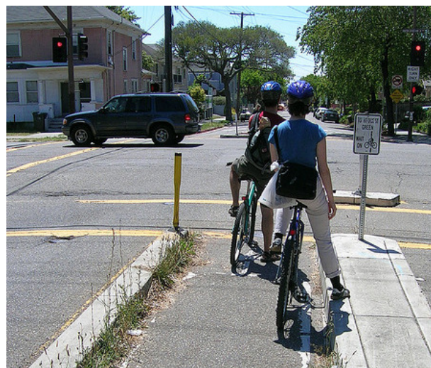
A bicycle detection system triggers a change in the traffic signal when a bicycle is detected.
