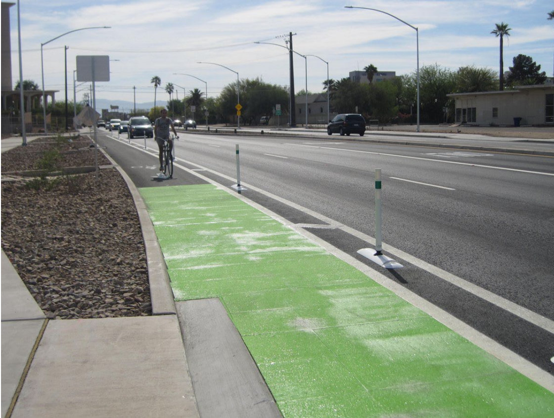
Image: Major Street with a Protected Bike Lan (Bollards Guideposts)
