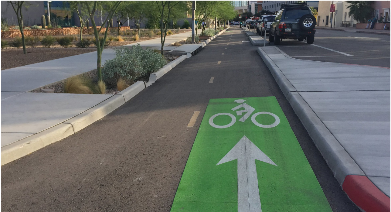
A two-way facility can accommodate bicyclists in two directions of travel.
