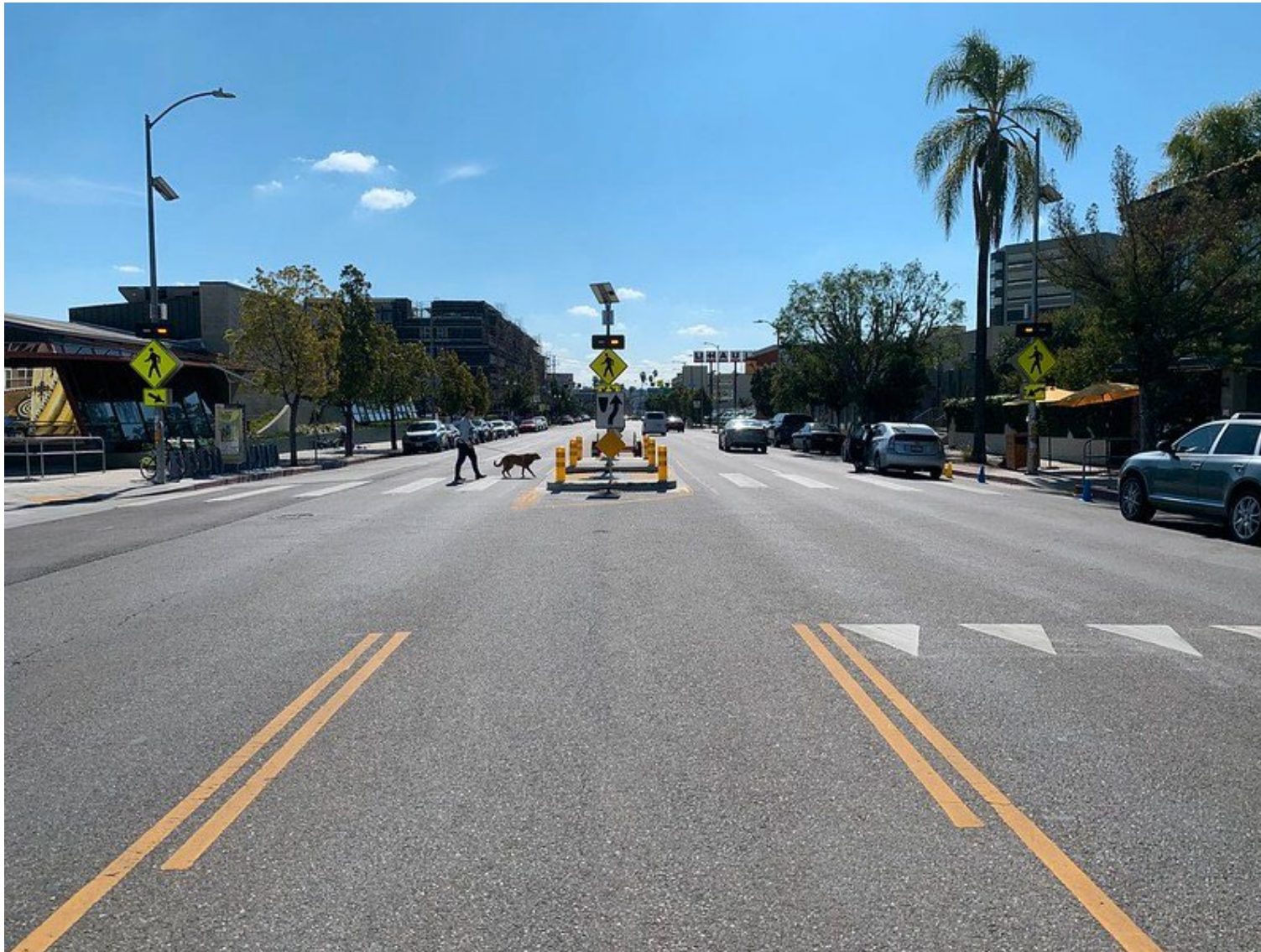
Image: Mid-block crossing with flashing beacon and island
