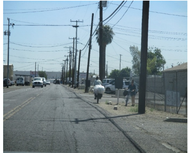
Figure 5-9: Missing sidewalk on Lincoln Street
