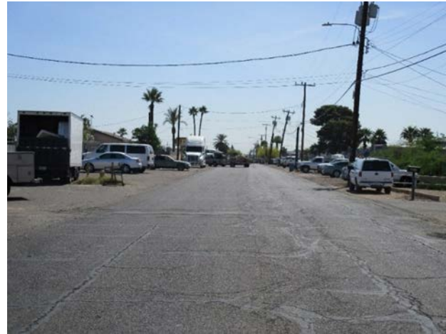
Figure 5-1: No sidewalks and vehicles on ROW
