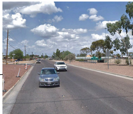
Lack of street lights
