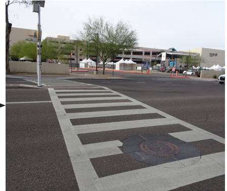
Example of a high-visibility crosswalk
