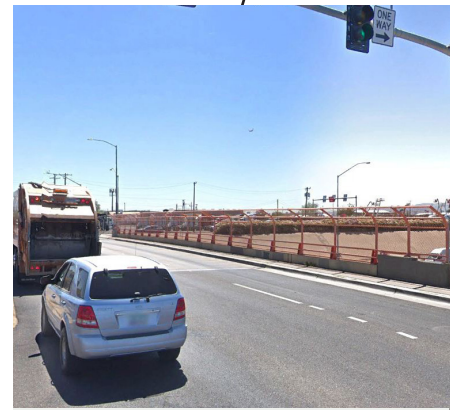
No protection from traffic for users crossing the bridge
