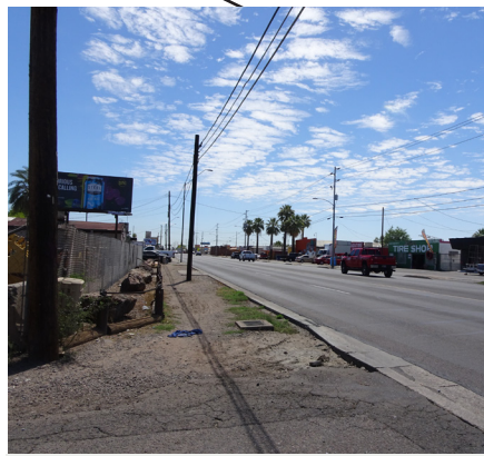
Gaps in sidewalk infrastructure
