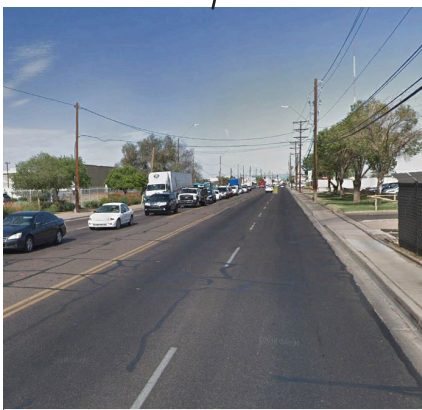
Lack of street lights
