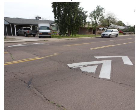
Example of speed hump
