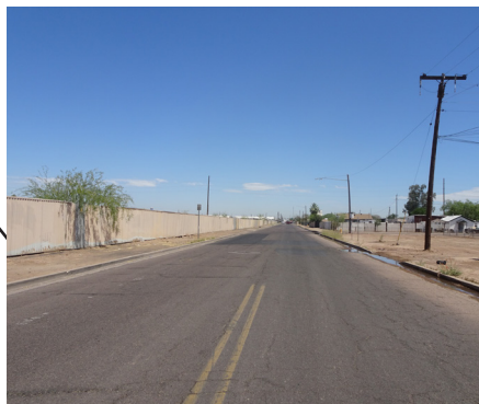
Lack of traffic calming measures to slow traffic
