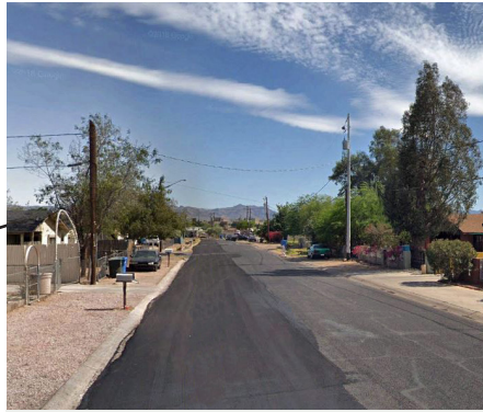
Lack of infrastructure to slow traffic
