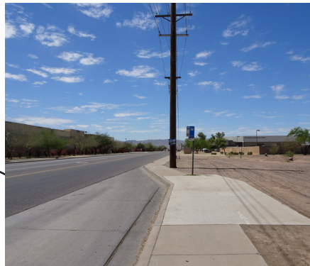
No north/south connection for bicyclists
