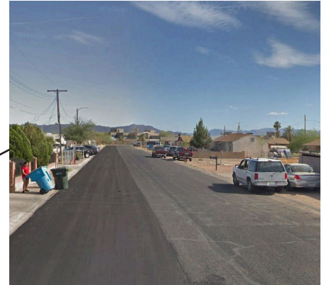
Gaps in sidewalk infrastructure
