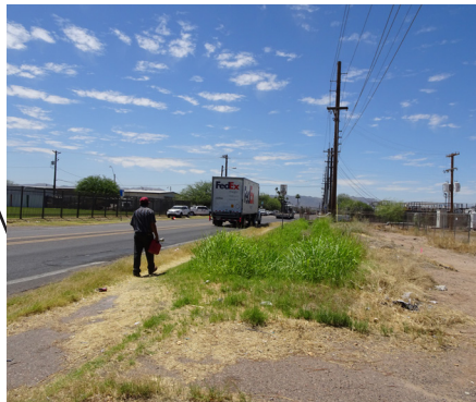
Gaps in sidewalk infrastructure
