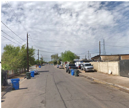
Gaps in sidewalk infrastructure
