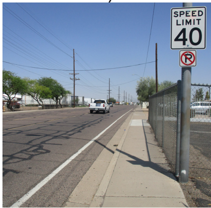
Lack of street lights
