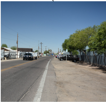
Gaps in sidewalk infrastructure
