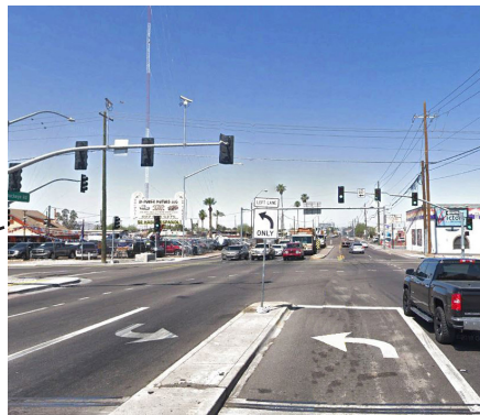
Lack of clearly marked crosswalk
