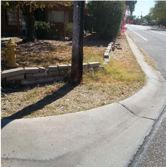
**Photo 18 - Mountable Curb & Gutter**
