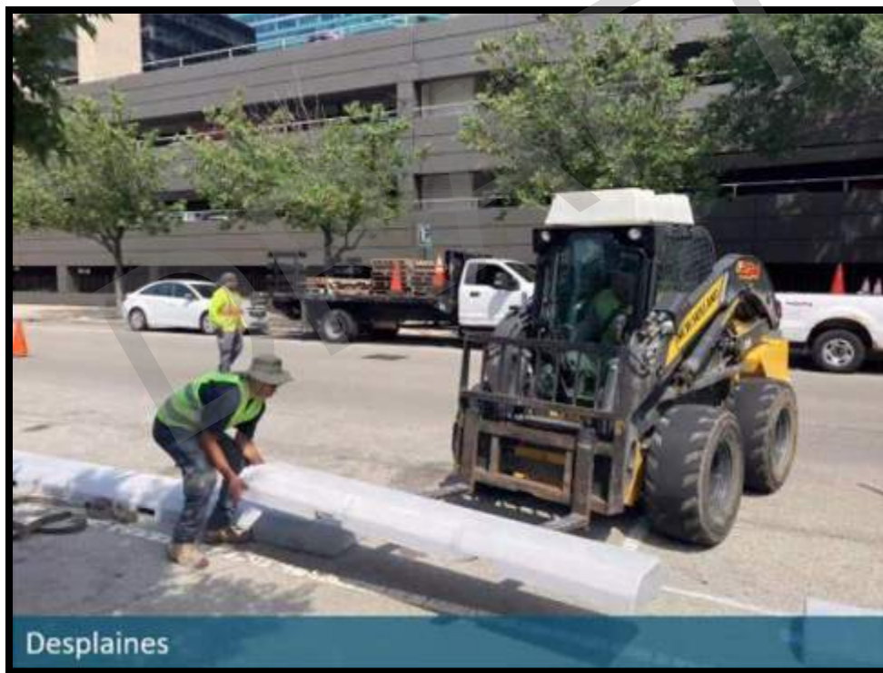
Figure 12 - Precast Concrete Curb Installation (Photo Courtesy of Chicago Department of Transportation)
