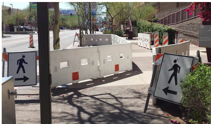
Figure 5 – Sidewalk Diversion Out-of-Street
