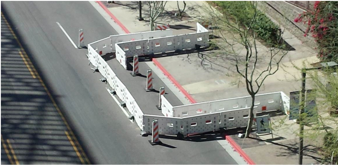
Figure 6 – Sidewalk Diversion In-Street
