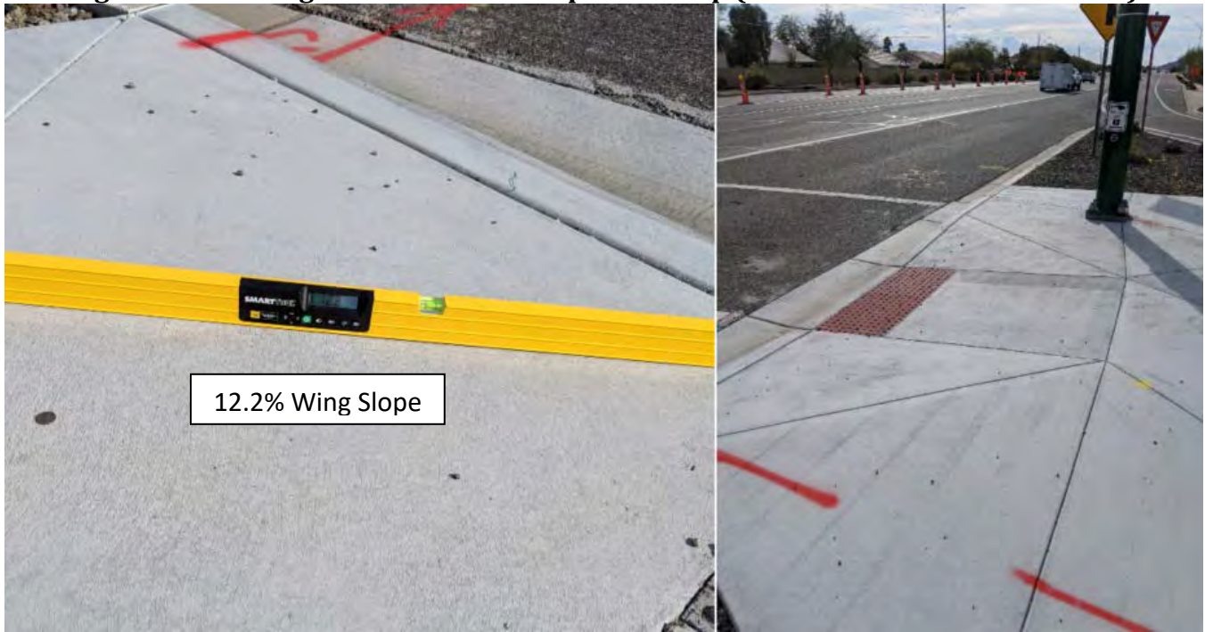
Figure 10: Existing PROWAG Non-Compliant Ramp (NW Corner of HVR & 55 th Ave)
