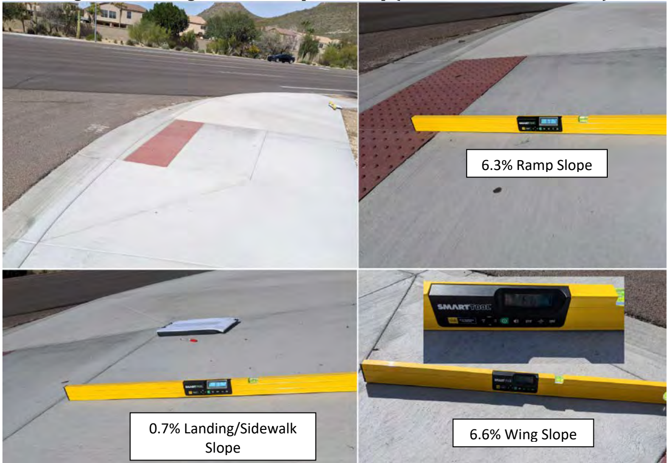
Figure 11: Existing PROWAG Compliant Ramp (SE Corner of HVR & 65 th Ave)
