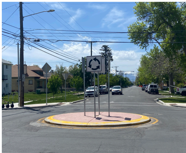
A traffic circle included in an intersection along a Bike Boulevard calms traffic since vehicles are forced to slow down. Photo credit: Alta
