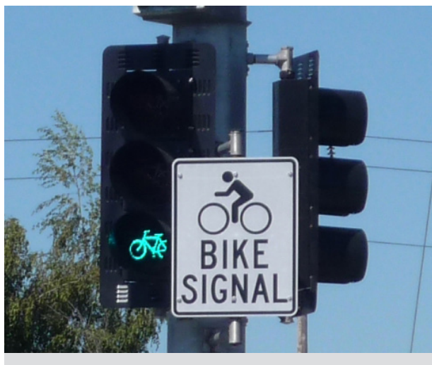
A bicycle signal head at a signalized crossing creates a protected phase for cyclists to safely navigate an intersection. Photo credit: TREC
