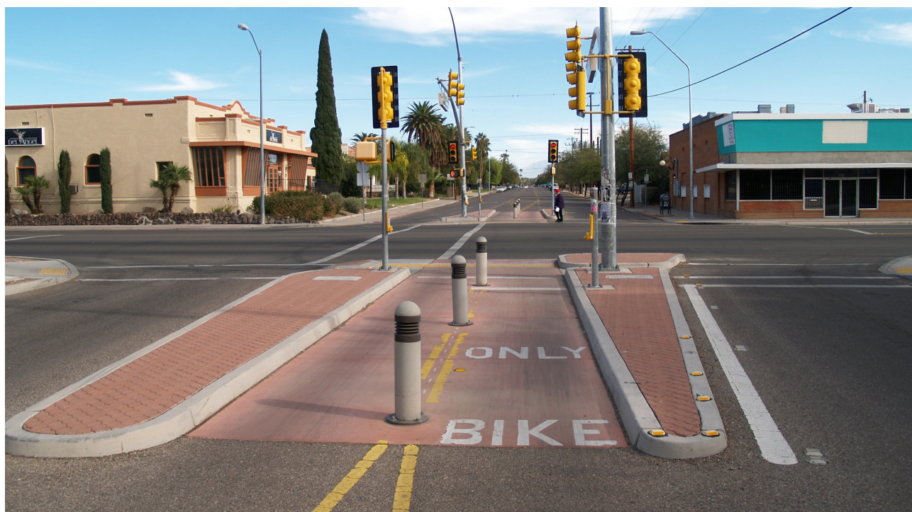
A Toucan signal in Tucson, AZ. Motorists must turn right onto Stone Avenue, the major roadway (from either direction). Bicyclists can turn left, right, or go straight. Bicyclists turning left or going straight can push a button to activate a green bicycle signal indication. Photo credit: Steven Vance.
