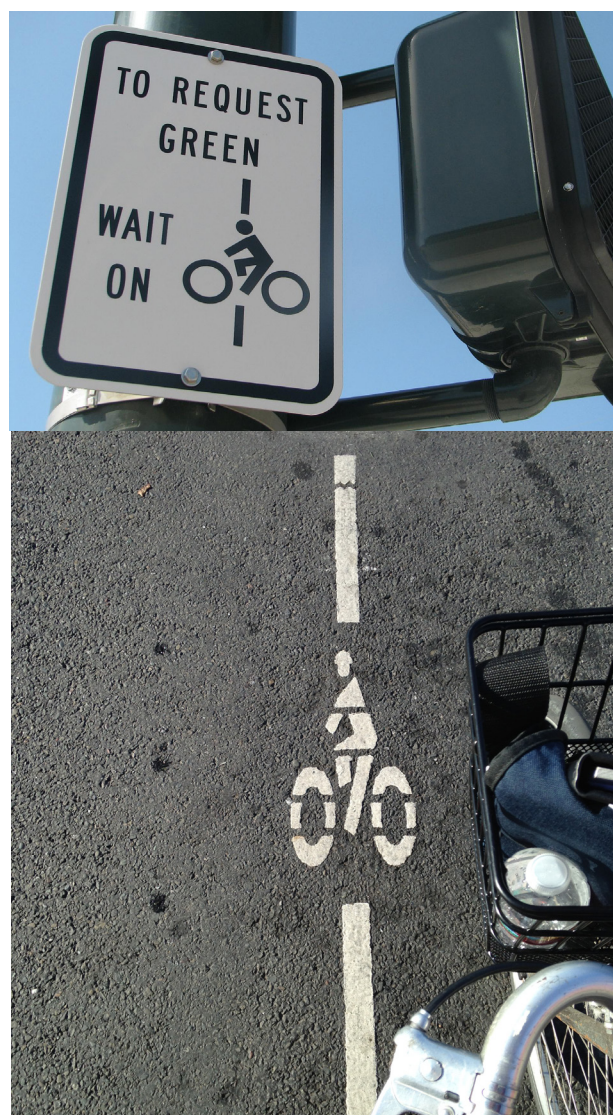
Pavement markings are paired with a sign to teach riders how to activate the bicycle loop detection
