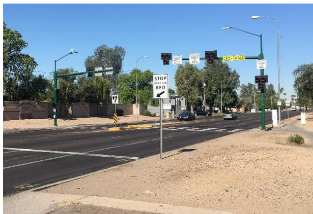
Existing HAWK on Thomas, west of 43 rd Ave.
