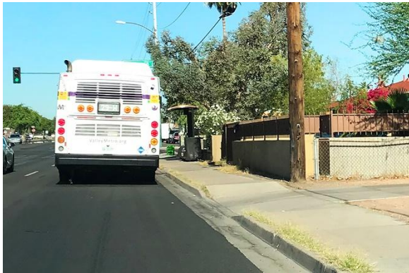
Existing Thomas Rd. sidewalk does not provide accessible route to bus stop.
