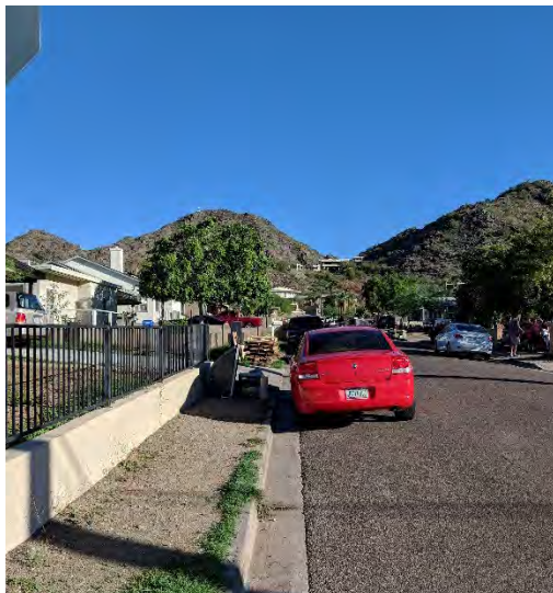
Figure 34: Sidewalk Gap on 3 rd Street north of Mountain View Road
