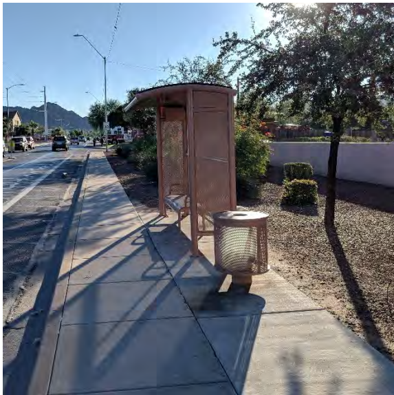
Figure 43: ADA Compliant Bust Stop on 12 th Street
