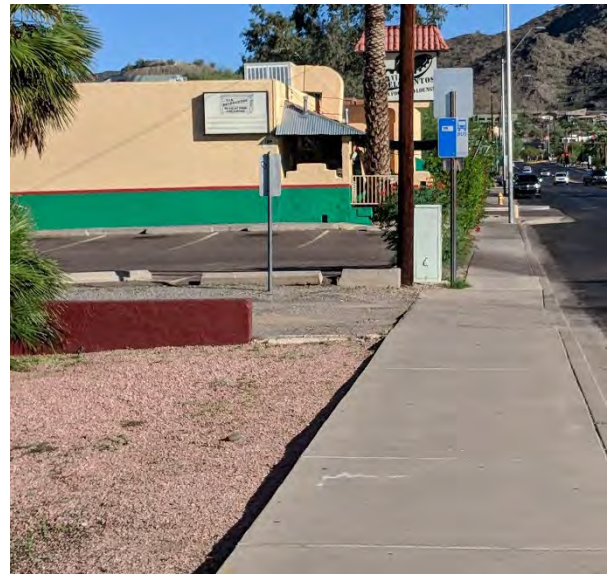
Figure 44: Non-ADA Compliant/Accessible Bust Stop on Central Avenue
