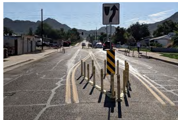
Figure 29: Temporary Traffic Calming
