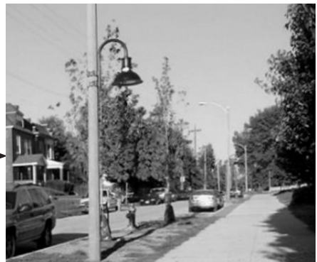
Example of street lights
