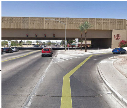
Narrow path under SR 202L and no barrier between pedestrians and vehicles
