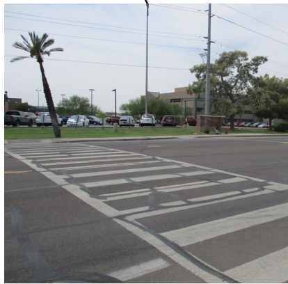
No signalized crossing at hospital
