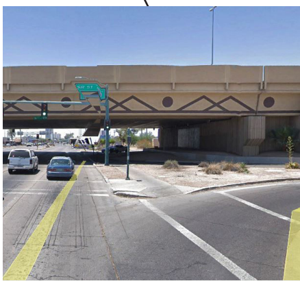
Narrow path under the SR 51 and no barrier between pedestrians and vehicles
