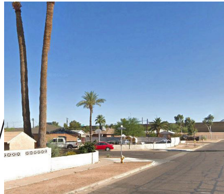
Gaps in sidewalk infrastructure
