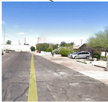
Gaps in sidewalk infrastructure
