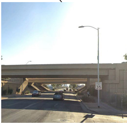
Narrow path under the I-10 and no barrier between pedestrians and vehicle
