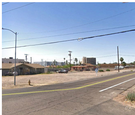
Gaps in sidewalk infrastructure
