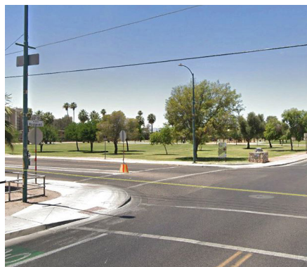
Lack of clearly marked crosswalk
