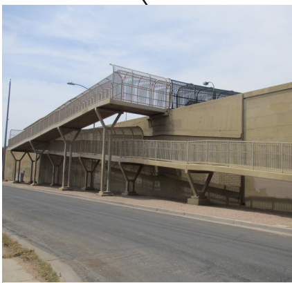
Pedestrian bridge lacks lighting and is a small enclosed walkway
