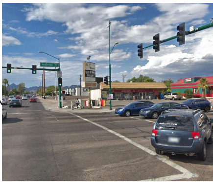
Lack of clearly marked crosswalk
