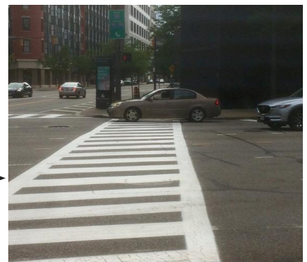
Example of a high-visibility crosswalk
