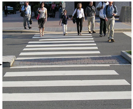
Example of a high-visibility crosswalk
