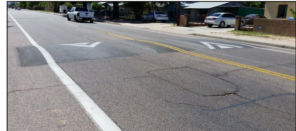
Figure 13: Example of Speed Cushion
