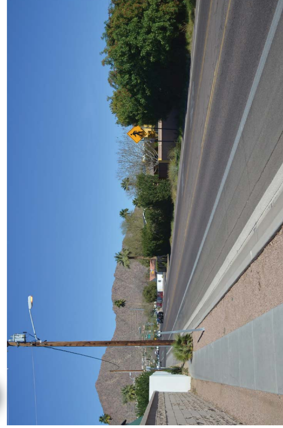
West Side of 56th Street at Flower Street Looking North along Noise Wall and Sidewalk
