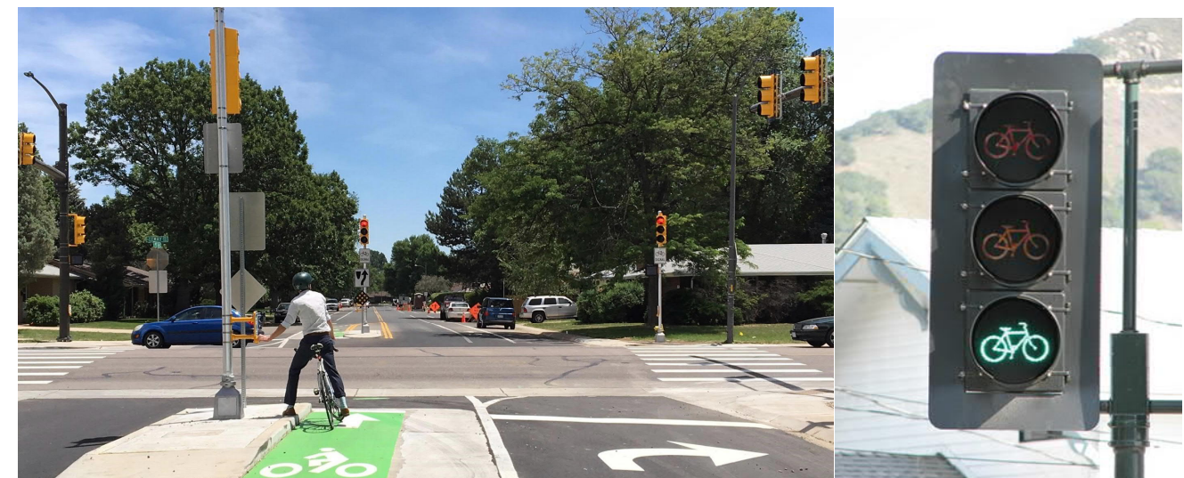
Figure 13: Bicycle Signal Application in Fort Collins, CO
