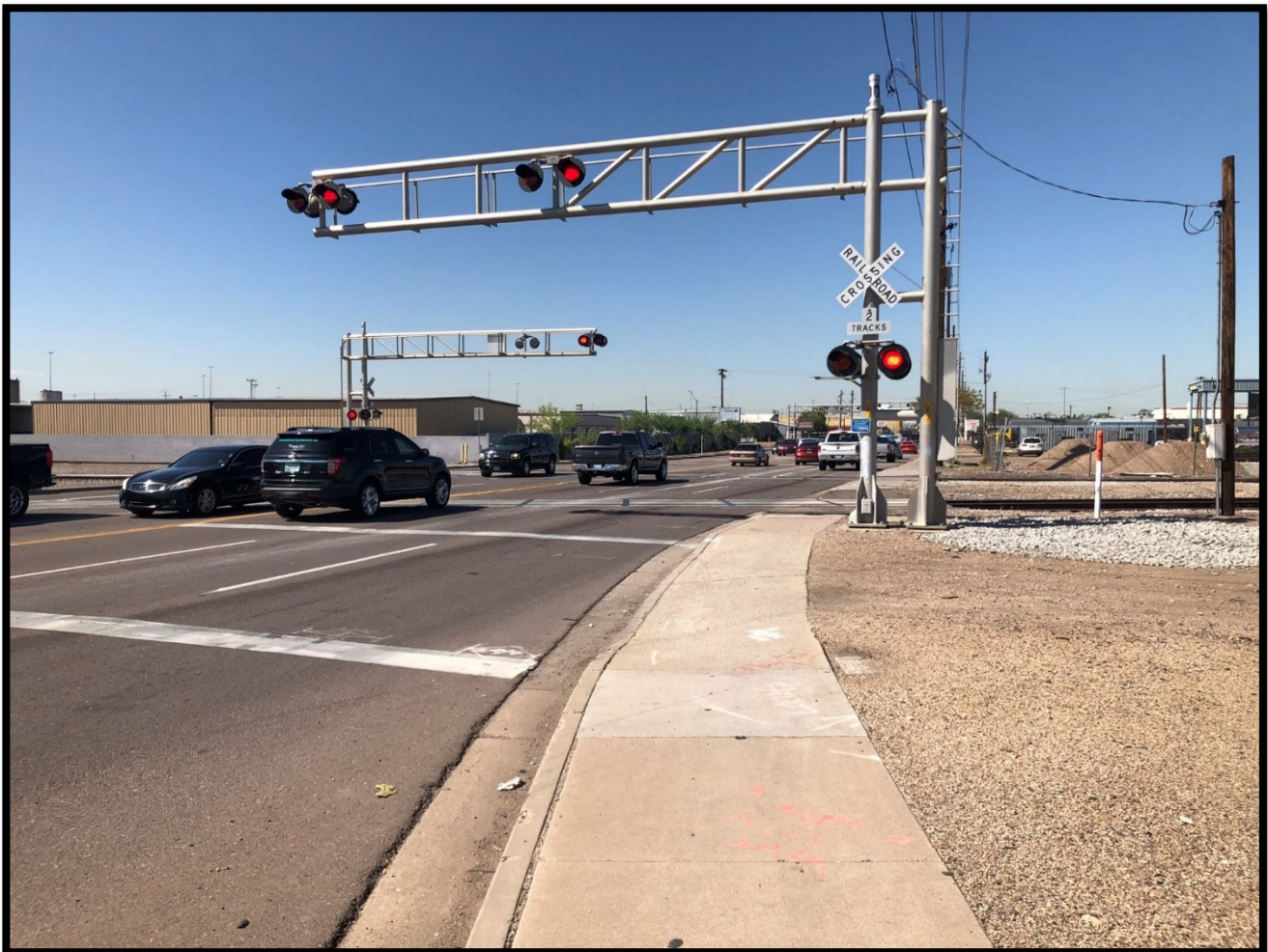
Figure 8 – Railroad Warning Devices at McDowell Road (looking west)
