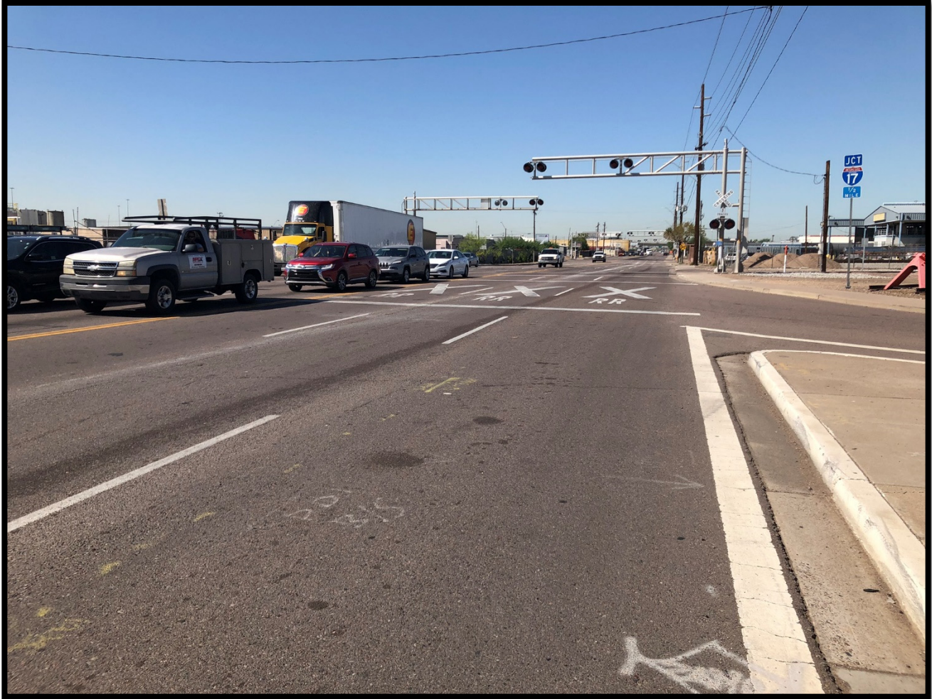
Figure 3 – McDowell Road (looking west)
