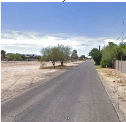
Gaps in sidewalk infrastructure
