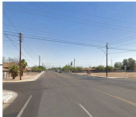
Lack of designated crossing
