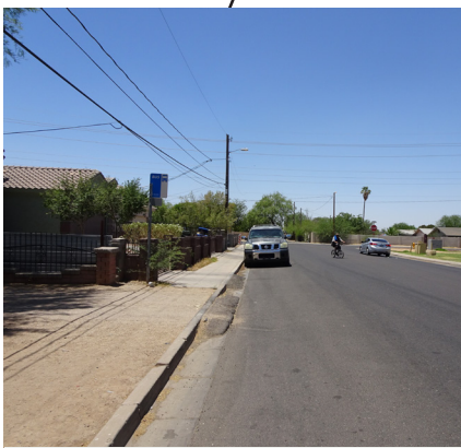
Gaps in sidewalk infrastructure
