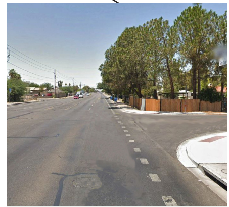
Lack of street lights
