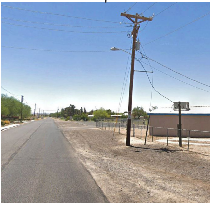
Gaps in sidewalk infrastructure
