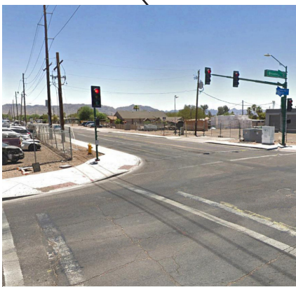
Lack of clearly marked crosswalks
