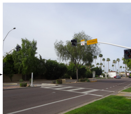
Example of mid-block crossing
