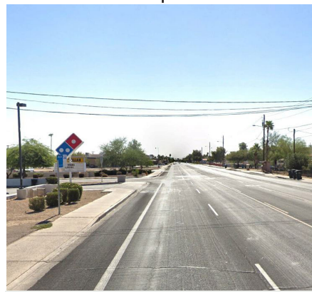
Lack of street lights
