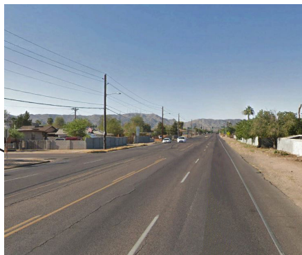
Lack of trees and street lights
