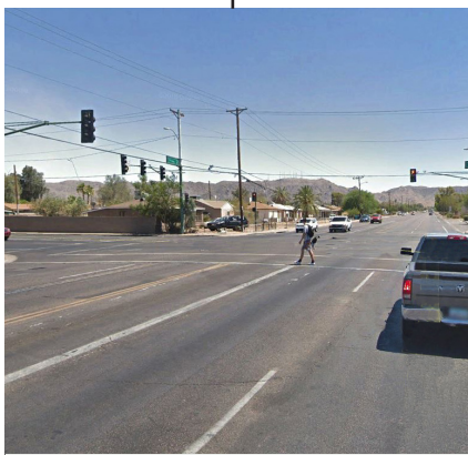
Lack of clearly marked crosswalks
