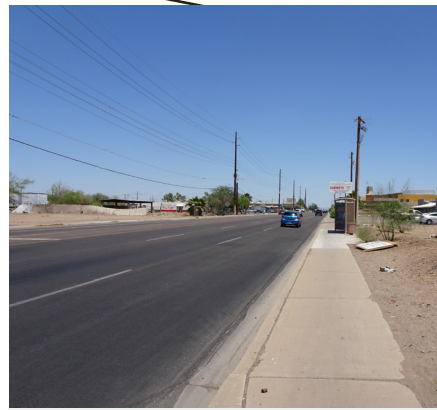
Lack of street lights
