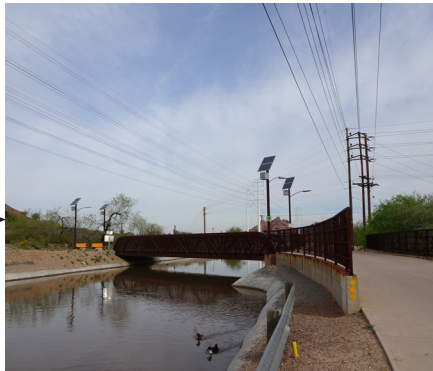
Example of a canal crossing
