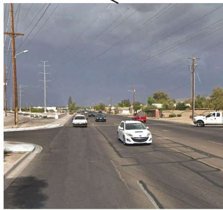
Lack of clearly marked crossing at Western Canal
