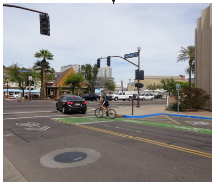
Example of intersection with bike box
