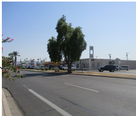
Lack of street lights
