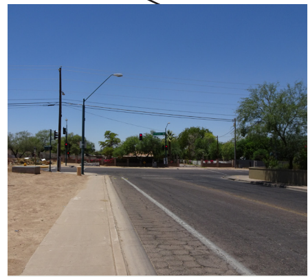
Gaps in bike lane infrastructure
