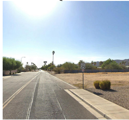
Lack of street lights
