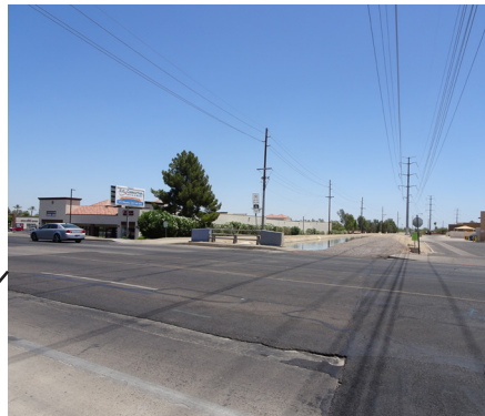
Lack of clearly marked crossing at Highline and Western Canal
