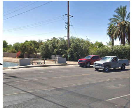
Example of bridge over canal
