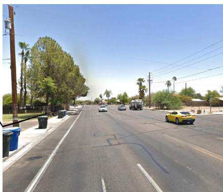
Lack of designated crossing
