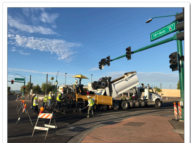
Asphalt paving at 19th Avenue and Camelback Road.
