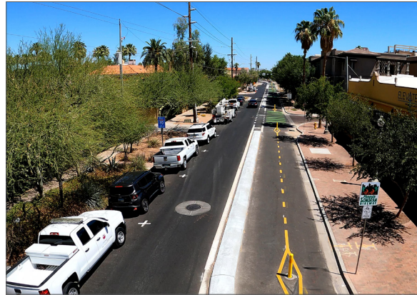
A protected bike lane reduces conflicts between bicycles and vehicles by providing physical separation between people biking and people driving.
