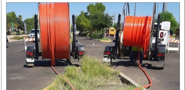
Integration of new fiber optic lines to assist traffic safety and operations.
