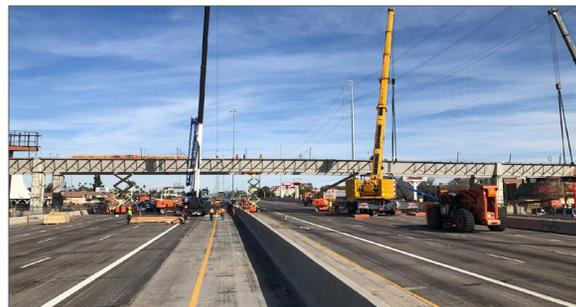
In March of this year construction crews completed bridge girder installation crossing over Interstate 17 for the Northwest Extension, Phase II.
