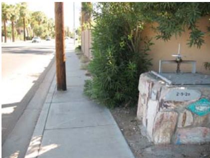
Photo: View South near Hoover Street., Utilities Limit Width of Pedestrian Clear Zone
