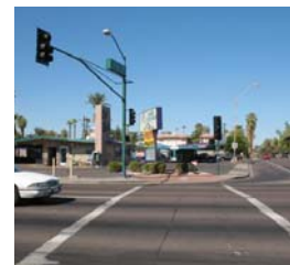
Photo: Examples of Sidewalk Ramps
