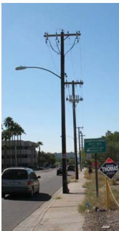
Photo: Existing power line pole obstructing sidewalk
