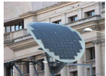
Photo: Solar Panel for Pedestrian Lighting
