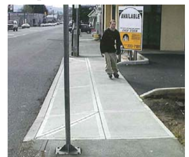
Photo: Driveway Crossing Example
