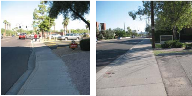
Photo: Example of Driveway Crossings with Excessive Cross Slope pedestrian circulation. When these are located in areas with planting strips, the sidewalk remains level, with driveway ramping up to sidewalk level in the planting strip width. However, when there is no planting strip, driveway crossings are incorporated into the sidewalk width and have excessive cross slopes which do not meet ADA standards.
