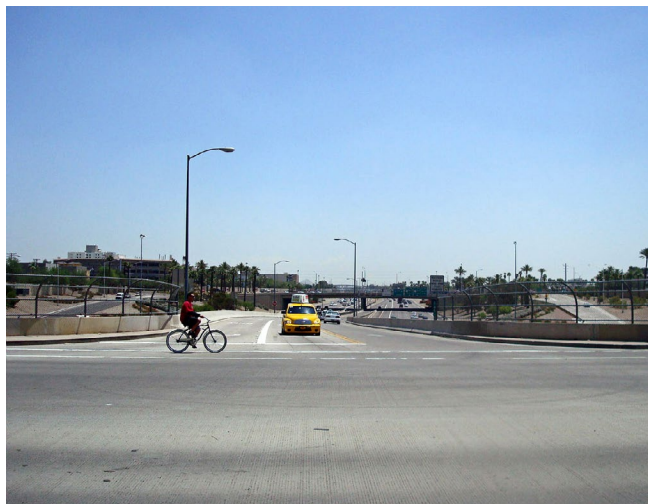
A bicyclist crosses the Interstate 10 overpass
