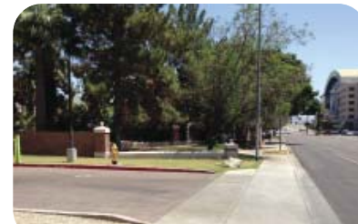
Photo No. 2 Children's Museum Driveway Bridge Landing Connection
