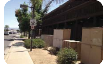
Photo No. 2 - 7th Street West Sidewalk Looking South
