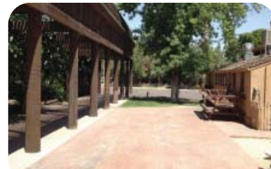
Photo No. 1 - Lath House Connection
