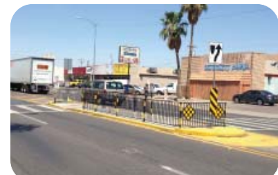
Photo No. 7 - Multi-stage Staggered Crossing at Van Buren St. Looking North West
