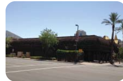
Photo No. 7 - Lath House Looking West from Children's Museum of Phoenix
