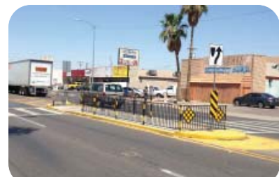
Photo No. 7 - Multi-stage Staggered Crossing at Van Buren St. Looking North West
