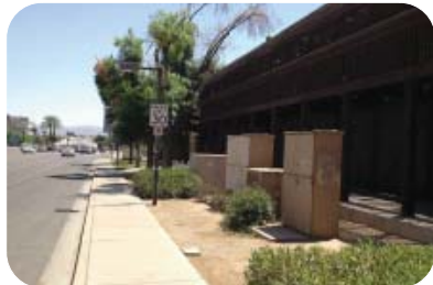
Photo No. 6 - Lath House - Utilities
