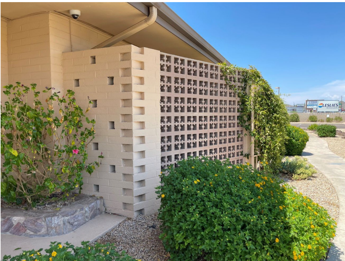
Offset screen wall on front façade of subject building, 2024.
