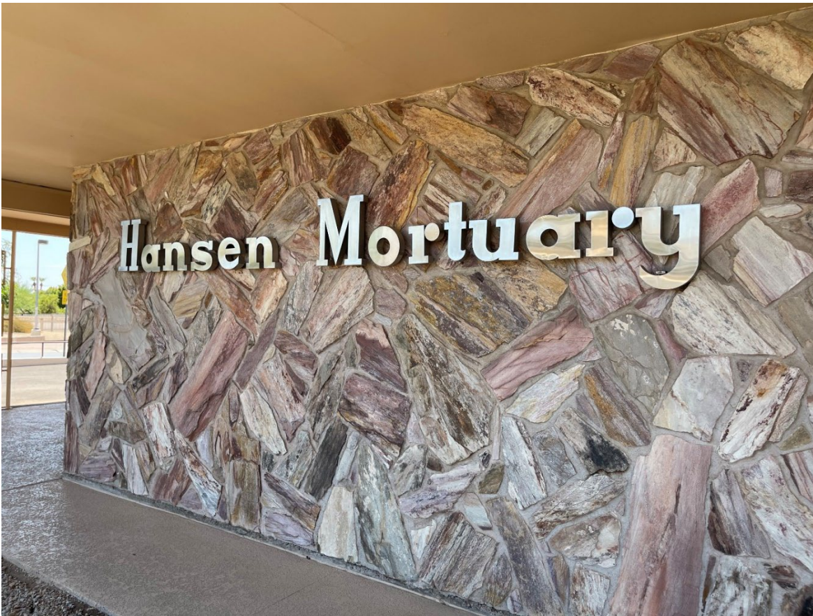
Native stone sheathed wall on front gable of subject building, 2024.
