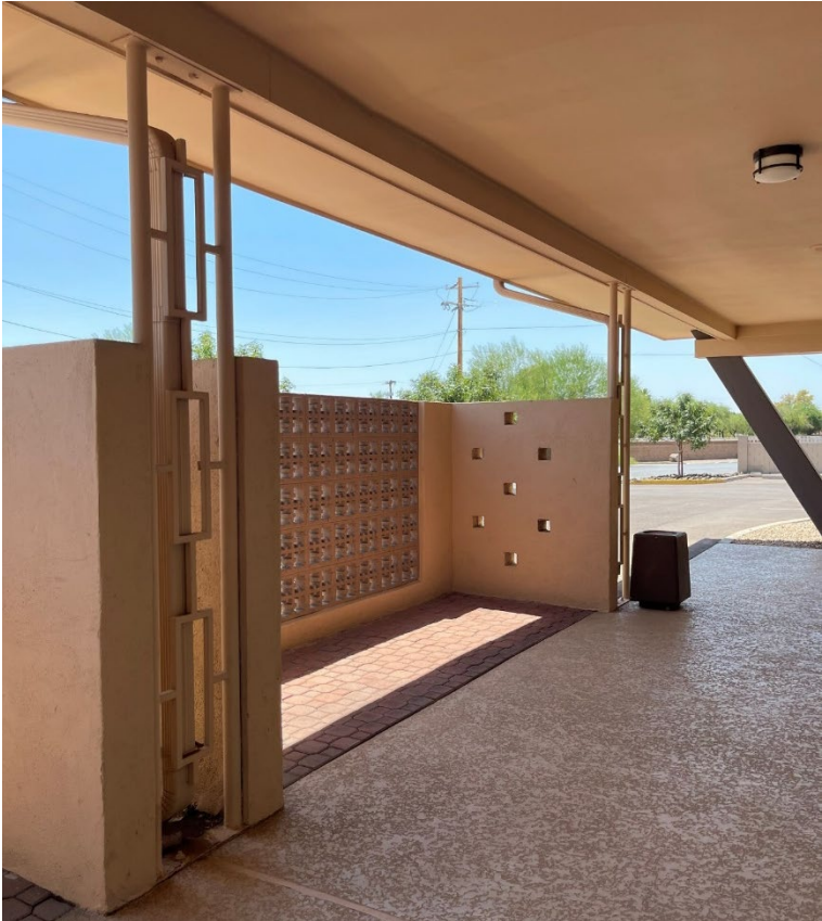
Decorative columnar breezeway supports, south façade of subject building, 2024.
