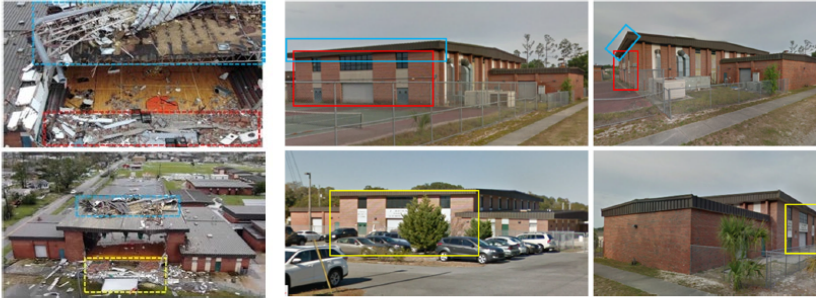
(a) After hurricane Michael
