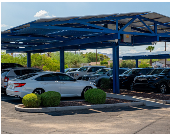
Dual-use of solar panels as shade structures for parking.
