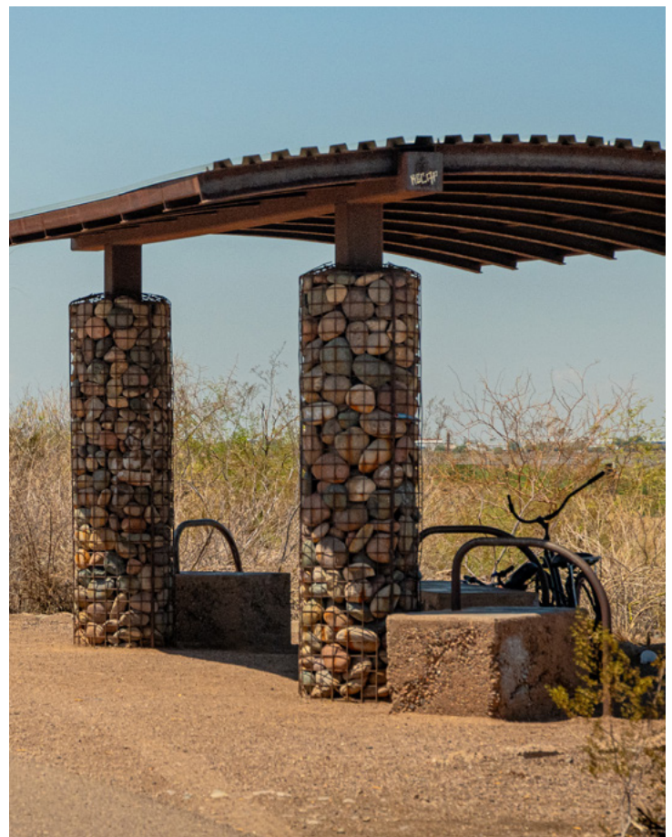
Use of natural materials, including caged rock and exposed concrete, to tie visually with the Rio.
