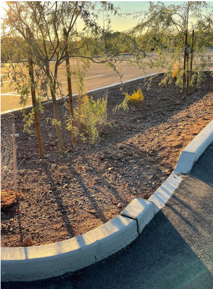
Parking lot curb opening for water infiltration.
