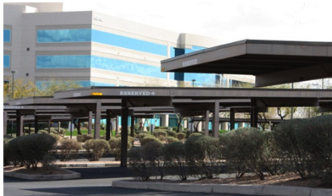
Figure 9. Covered parking (Source: Kimpel & Butler)
