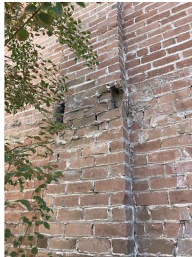
**DETERIORATED BRICK PILASTER (WEST ELEVATION)**
