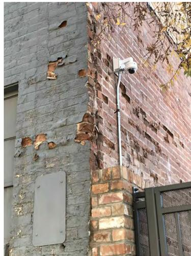
**DETERIORATED BRICK AT CORNER**
