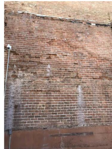
**DETERIORATED BRICK (WEST ELEVATION)**
