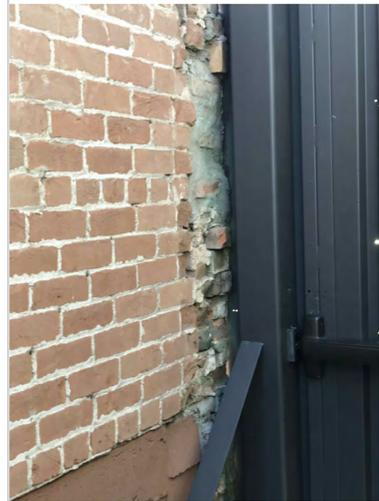
**DETERIORATED BRICK AT CORNER**
