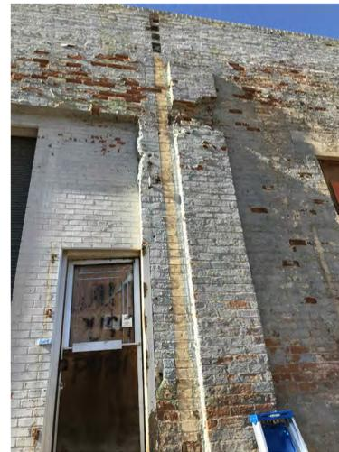
**PAINTED/DETERIORATED BRICK (EAST ELEVATION)**
