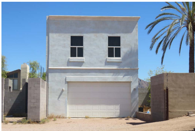
2-story Garage- looking north
