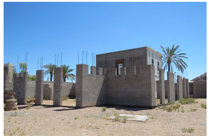
Partially-built structure (to be removed)- looking northeast
