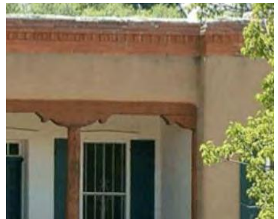
In some instances, greater detail may be given to building components such as the design of beams, and facade elements such as shutters or molding may be used.
