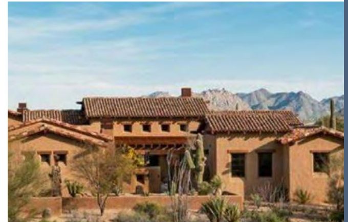
The design imagery shows stucco, sloped tile roof, recessed openings, and building and site layout/orientation to preserve building adjacency/proximity too open space between and connectivity to surrounding buildings
