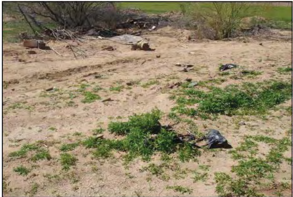
8 MINOR DEBRIS AT SOUTHWEST CORNER OF SITE
