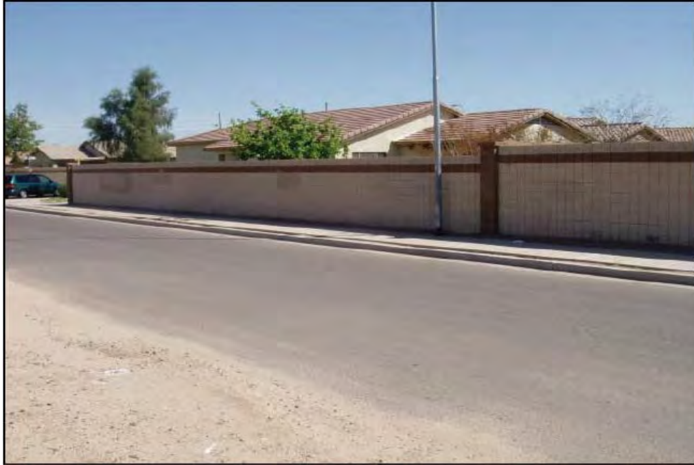
13 ADJACENT PROPERTY EAST OF SITE
