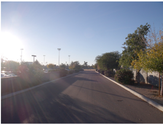
View 8 Facing west
