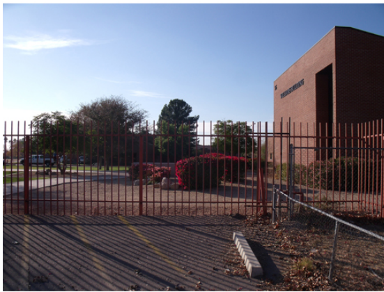
View 36 Facing west
