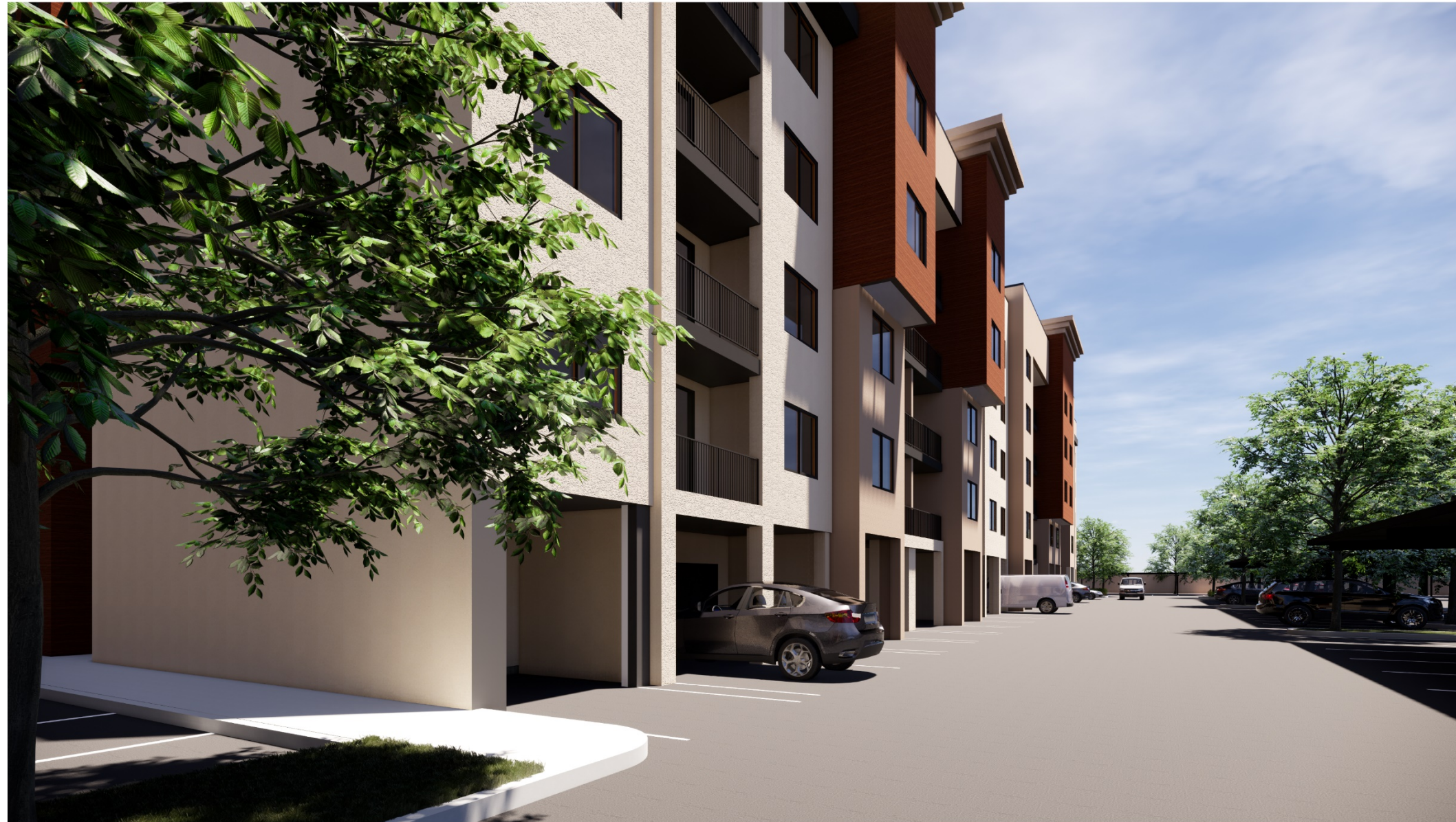
VIEW OF EAST BUILDING LOOKING SOUTH
