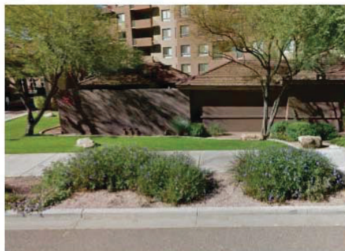
16. SOUTHWEST CORNER LOOKING WEST
