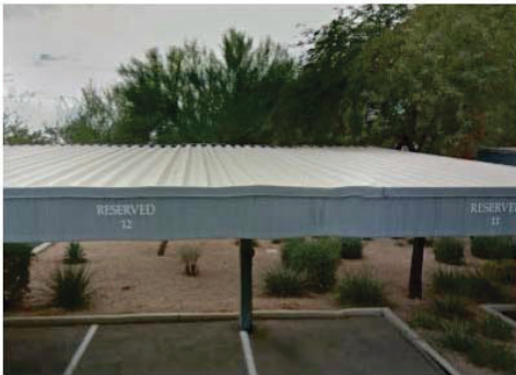
7. EAST MID-POINT LOOKING SOUTH
