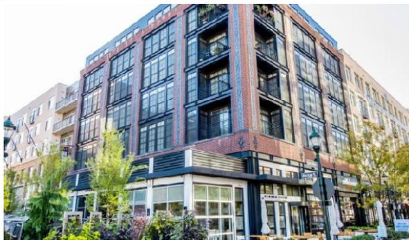
5.2f.3 In addition to window glazing, up to three primary materials are permitted for individual tenant storefronts. Provide quality, durable materials that have a natural appearance for all tenant storefronts. Metal, stone, brick, cast stone, concrete, and plaster are recommended materials.
