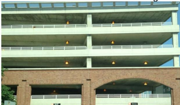
5.3.4 Exterior elevations of parking structures should have an open-air design to allow for natural visibility to and from adjacent streets and nearby buildings. Sheer panels are permitted.
