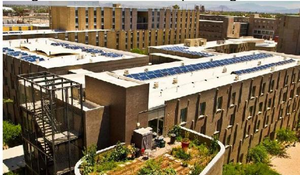
5.2d.4 Rooftop photovoltaic solar panel systems are encouraged for both buildings and parking garages, but these systems shall be set back a minimum of 25 feet from the parapet and should have a maximum height of 12 feet.
