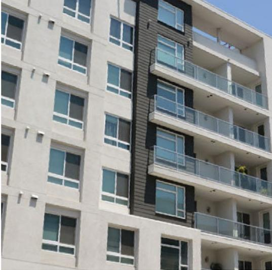
5.4b.2 Where more than one material is used in a facade, heavier materials such as stone/brick veneer should be located below lighter materials such as stucco. The change in material should occur along a horizontal line at the floor level.
