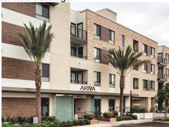
5.4a.2 Mortar joints shall complement the masonry color. Masonry units shall have butt joints at outside corners with a minimum 4-inch overlap. Bricks may be coursed in common, running bond, herringbone, Flemish, basket weave, or horizontal patterns.
