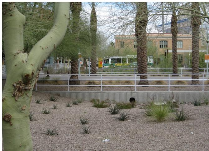
This investment contributes to permeability, and can be used to promote cooling. In general, properly designed and constructed retention cells achieve excellent removal of heavy metals, moderate storm water discharge, enhance wildlife habitats, and act as windbreaks and noise absorption.
