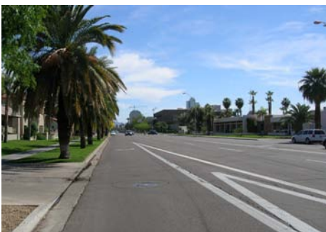
Existing bike lanes on 3rd Street 3rd Street near McDowell Road.
