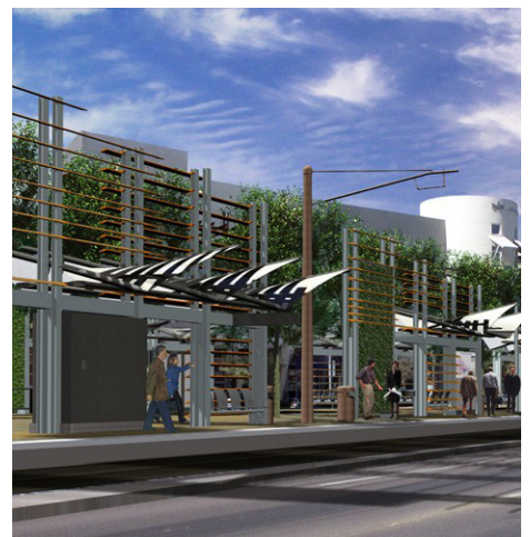
Light Rail Station at Central Avenue and Roosevelt Street
