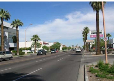
Some segments of east-west streets may experience congestion because there are a limited number of through-streets that run east-west. (McDowell Street between 3rd and 5th streets)
