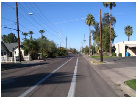
Existing bicycle lanes on 3rd Avenue near Willetta Street.
