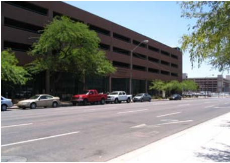
An existing parking structure in Downtown (Jefferson Street at 4th Avenue)
