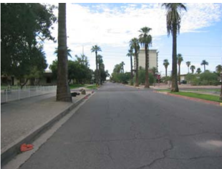
Downtown Local Street – McKinley Street
