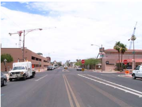
The 1st Street right-of-way is 100 feet. There is room to add either a linear park in a median, or extensive landscaping and wide sidewalks on both sides of the street.
