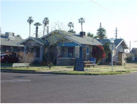
Adaptive reuse of a bungalow at 5th and Garfield Streets
