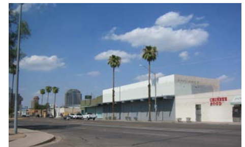
Commercial, institutional, and industrial uses are located along Central Avenue.
