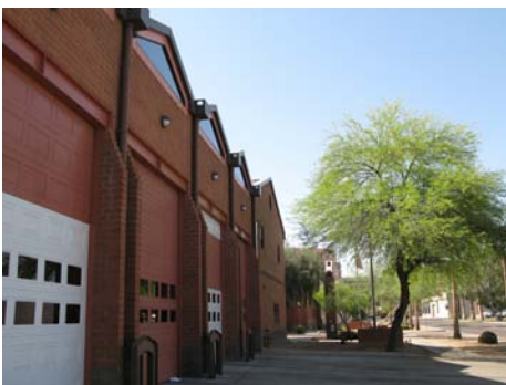
Fire station on 4th Avenue north of Van Buren
