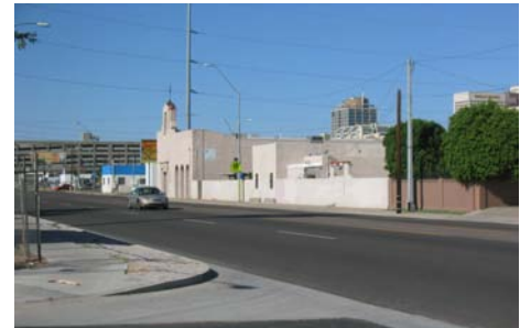
The Grant and Lincoln corridor will transition from a strictly industrial area to a commercial area.
