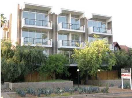
Multi-family development near Willetta Street and 5th Street
