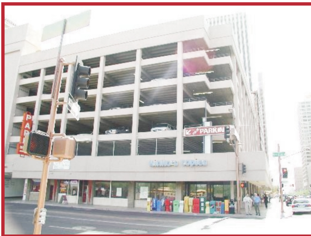
FIGURE 11 - Parking Structure with Non-parking Uses on the Ground Level
