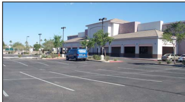
Vacant supermarket anchor store at 19 th Avenue and Greenway Road
