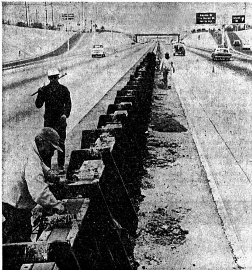
Figure 6: SAFETY BARRIER —Workmen for William Pulice Contractors install frames near Grant Street underpass for a concrete median-barrier that will run down the center of Black Canyon Freeway from Buckeye Road to Arizona Canal. The 32-inch-high buffer, designed to prevent head-on collisions, is scheduled for completion in July. (Circa 1970's)
