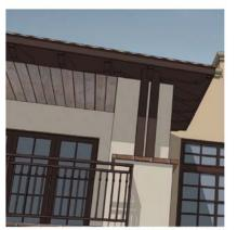
BALCONY WITH ROOFED WITH IRON DUEL POST WITH SPANISH TILE BASE; DECK CEILING WITH WOOD TILE TEXTURE
